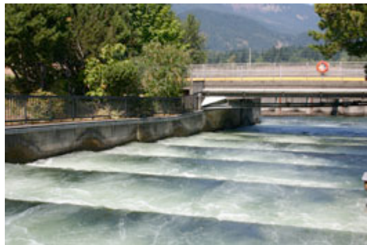
Fish Ladder at the Bonneville Dam on the Columbia River Separating Washington and Oregon
